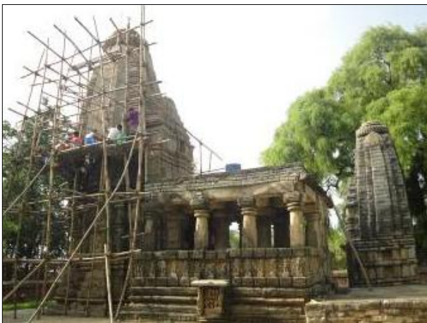
42-43. Mahadeva and Surya Temple, Narayanpur, Chhattisgarh: Removal of biological agencies from the outer surface
