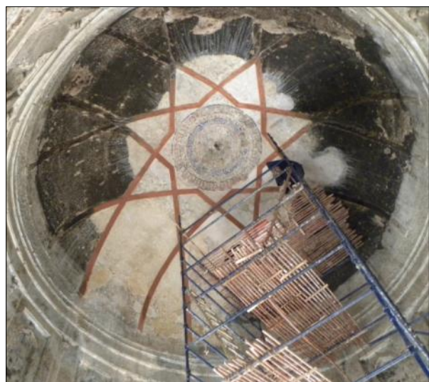
59. Bara Lao Ka Gumbad, Vasant Vihar, Delhi: Algae/ Lichens growth due to dampness
