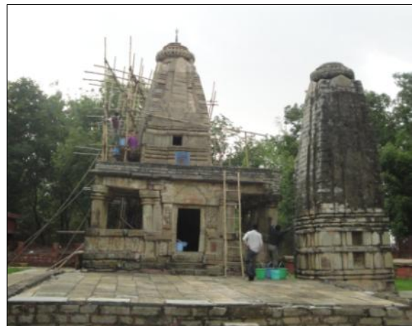
42-43. Mahadeva and Surya Temple, Narayanpur, Chhattisgarh: Removal of biological agencies from the outer surface
