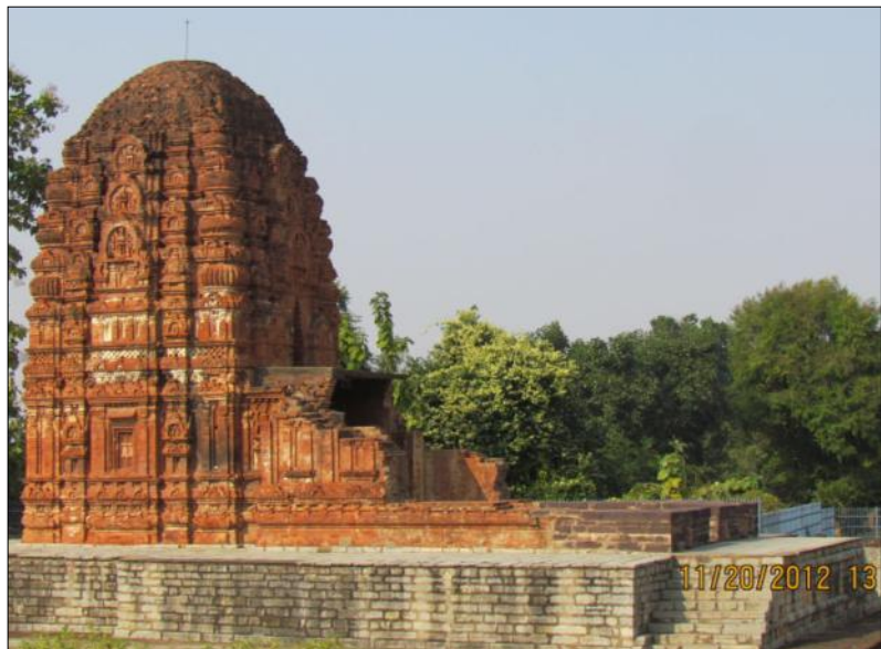
2. Lakshman Temple, Sirpur: A brick structure
