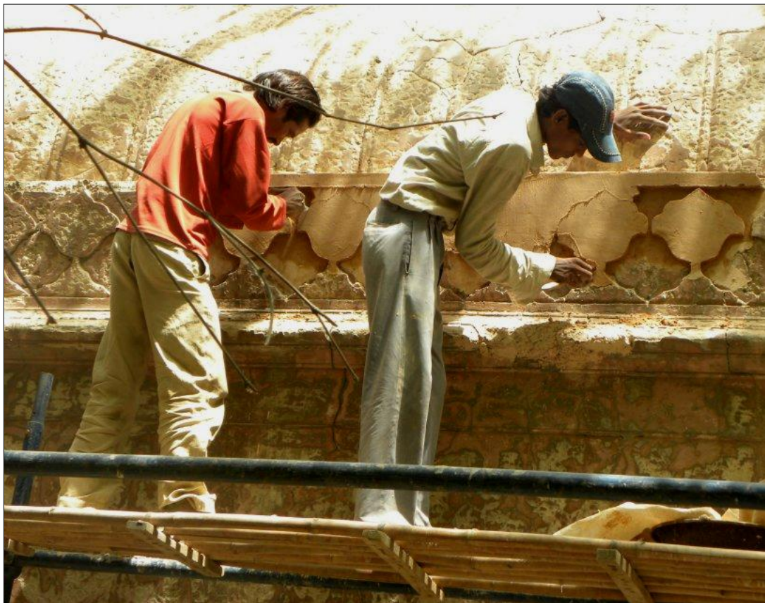
65. Unknown Mosque, New Delhi: Restoration of kangoora design using lime mortar
