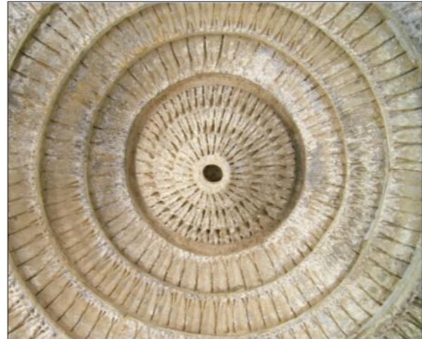
25. Munsar Tank, Viramgam: Ceiling of mandapa showing Sahatrakamala design
