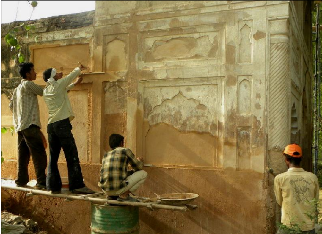
64. Gateway, New Delhi: Restoration of missing ornamental lime plaster
