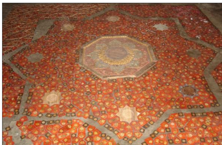
50. Maharaja Ranjit Singh Summer Palace Museum, Amritsar: Ceiling assembled on ground after dismantling
