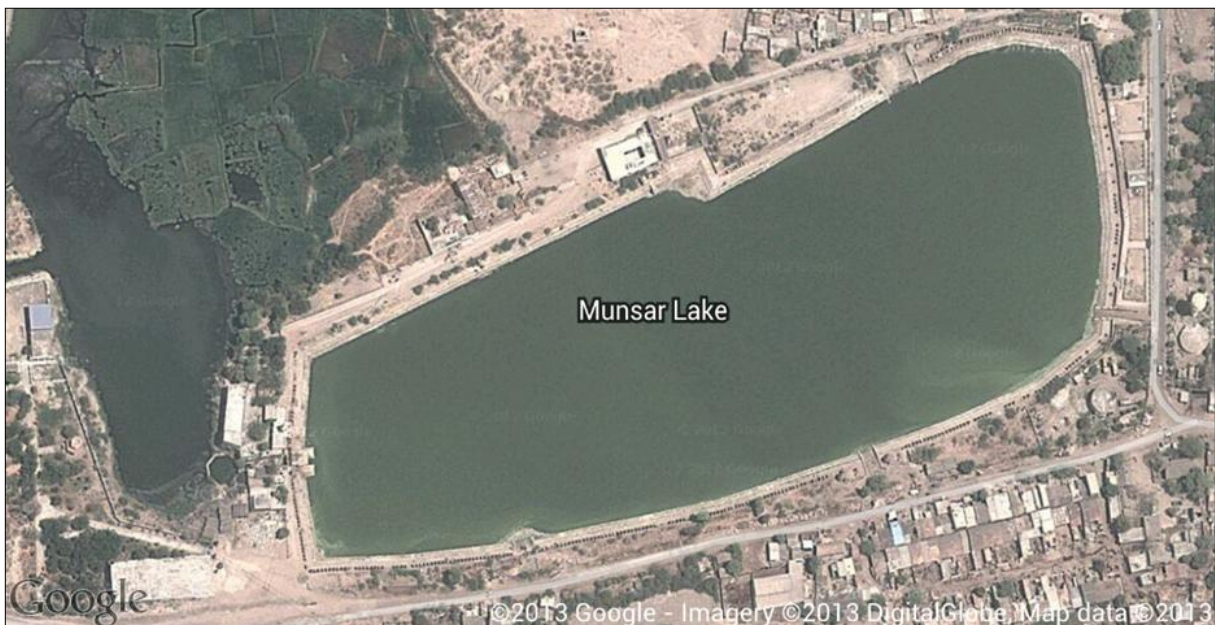
17. Munsar tank, Viramgam: Google Imagery (Source: Google Earth)
